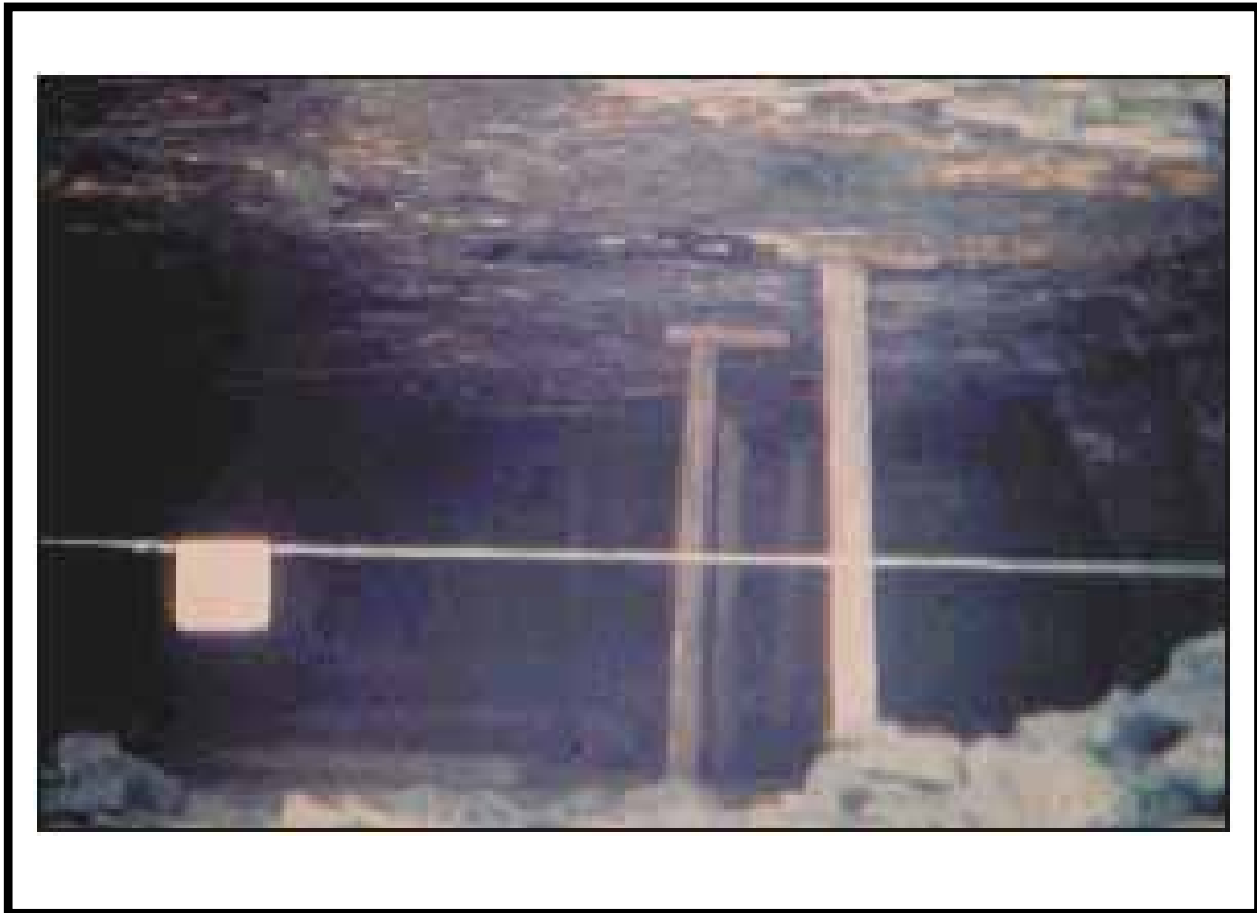
Figure 4 The conditions of the underground board and pillar workings
