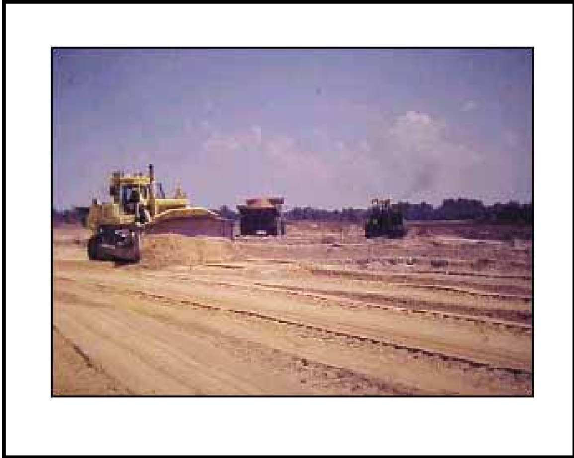
Figure 21 The leveled spoils with sand being placed.
